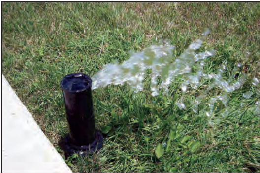
Figure 6 - Sprinkler hit by lawnmower.
