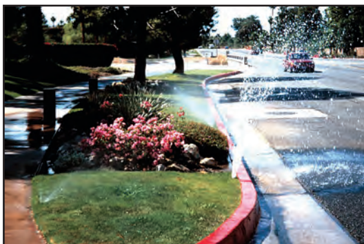
Figure 1 - Broken sprinkler floods street and hardscape causing damage.
