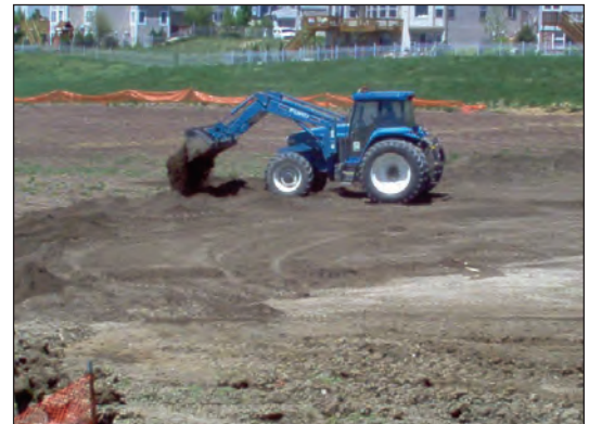
Figure 34 - Subgrade installation of Techline CV with soil being laid over a grid layout. Note how the loader is moving parallel to the driplines to minimize the rows from shifting.
