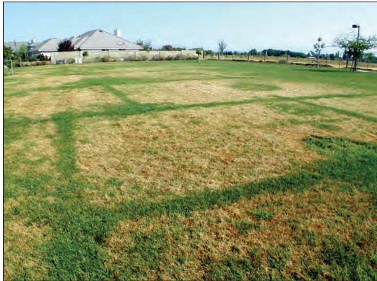
Figure 33 - Example of a sprinkler system where the trenches were not properly compacted after the PVC pipe was installed.
