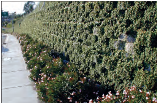
Figure 24 - Examples of pocket walls irrigated with Netafim Dripline.
