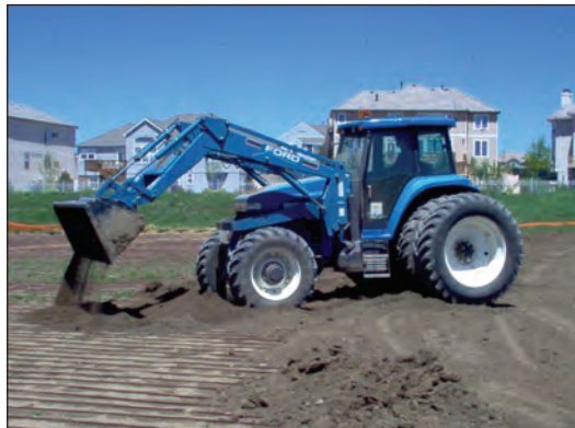
Figure 34 - Subgrade installation of Techline CV with soil being laid over a grid layout. Note how the loader is moving parallel to the driplines to minimize the rows from shifting.
