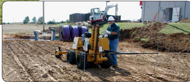
Figure 17 - MB-40 Does Not Disturb the Grade. Even in bare dirt.
