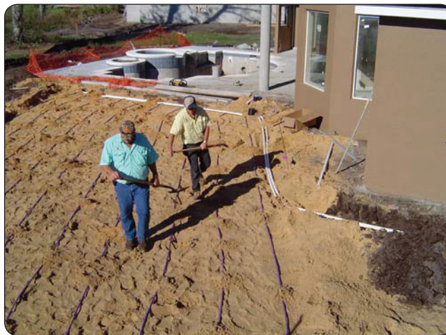
Figure 19 - "Drip and Fill" Technique.
