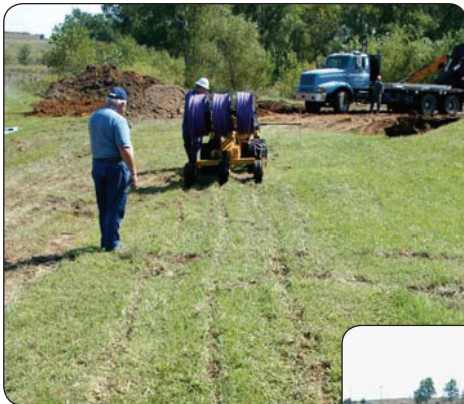
Figure 16 - MB-40 Minimizes Damage to Existing Landscape. Thanks to its unique design, the MB-40 quickly rake-up of this area, the rows virtually disappear.
