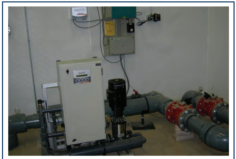
FIGURE 4. Fertilizer injection system
