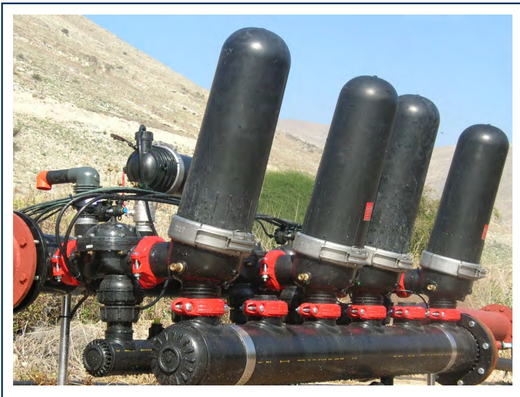
FIGURE 2. Automatic Self-Cleaning Disc Filters
