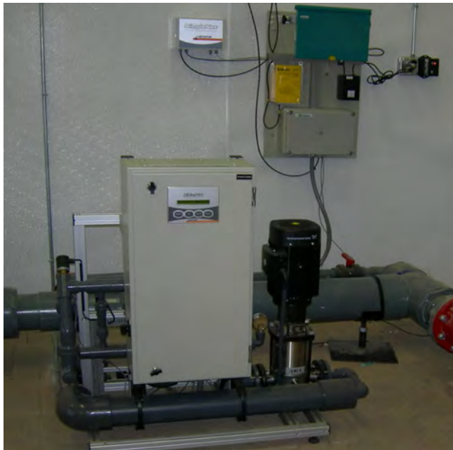
Figure 2.4. A Netafim fertilizer injection and irrigation control system. Flow meters are located on the right a pressure gauge is visible on the left.
