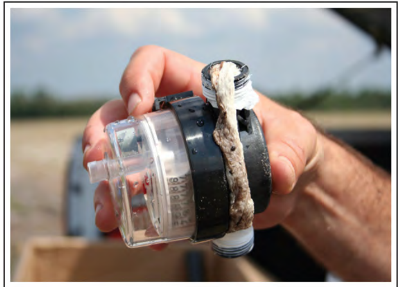
Figure 7.2. Filamentous sulfur slime completely clogging a small water meter.
