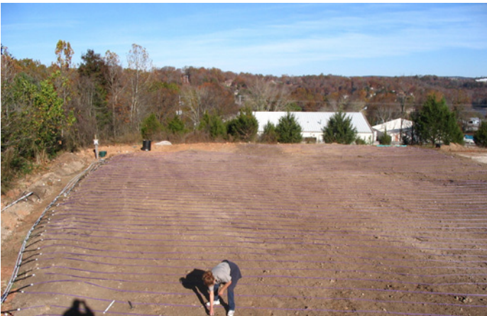
Before bringing soil in to cover the dripperline, a crew member ensures that the rows are equally spaced and held in place with soil staples.
