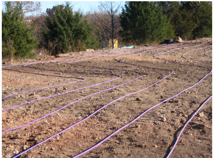
The flexibility of Netafim Bioline is an important feature. It allows the designer to match the dripperline to the shape of the dispersal areas with ease.
