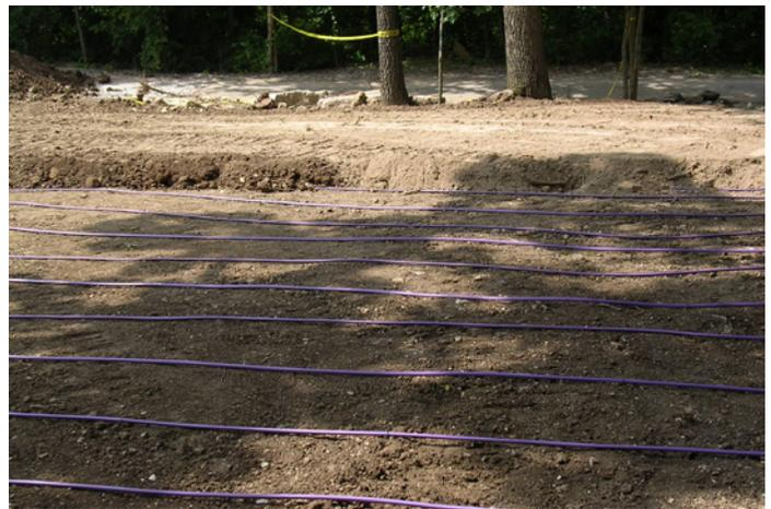
6" soil lifts were used to cover the Bioline in the drip fill. This technique is referred to as 'drip and fill'.
