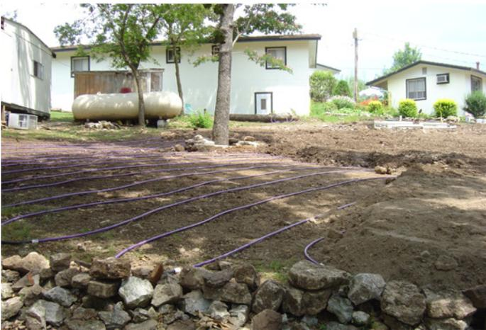
As shown above, when laying the dripperline on a slope, it is recommended that the dripperline be laid perpendicular to slope.
