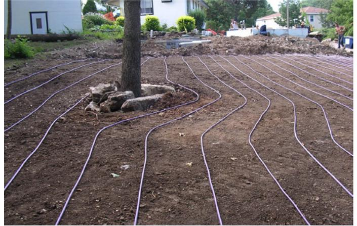
Here is an excellent example of the flexibility of Bioline drip dispersal tubing. It easily allows the designer and installer to adapt to the shape of the dispersal field.
