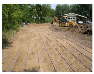
Once the dripperline was laid out, the contractor used a loader to add topsoil over the dripperline. This technique allowed the operator to keep heavy equipment from rolling over the dripperline.
