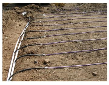
A lack of existing soil required that additional fill be brought in before the Netafim Bioline could be laid out. Notice the use of flex PVC to transition from the supply and return headers up to the dripperline laterals. This helps to protect the dripperline from damage in poor soils as well as preventing drippers from being placed outside the boundary of the drip field.
