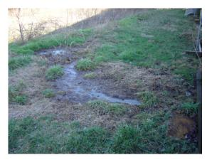
Prior to system renovation, the sewer line was dumping raw sewage directly on the ground.
