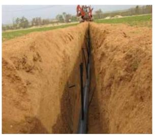
Get into the trench and use a narrow spade to clear the area between the dripline outlet and the trench wall. This will expose 4" to 8" of the buried dripline.
