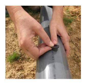
Insert riser - it is recommended to wet the insertion tooth to reduce friction. Insertion will be done by slight movements exerting pressure onto the submain pipe and done while the PVC pipe is outside the trench.
