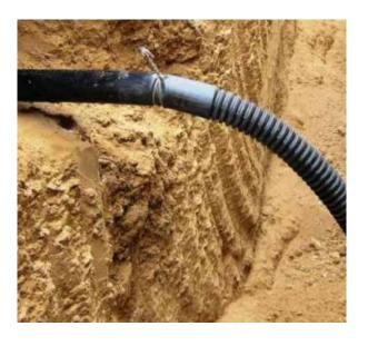
Lock the dripline onto the inserted riser using double loop stainless steel wire ties and tighten using a specially designed wire tie tool. Wire ties and tool not sold by Netafim.
