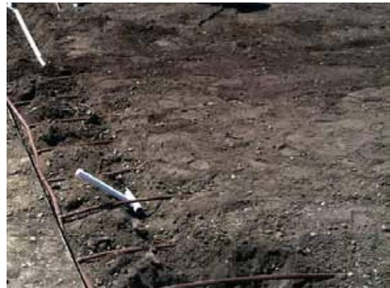
Netafim Techline CV Dripline is installed 4" below the soil and secured with 6" soil staples every 4' along the dripline.
