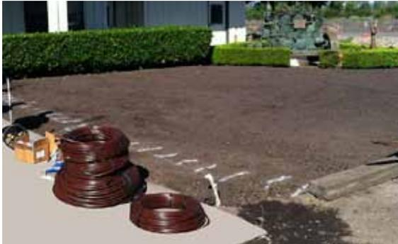
Marked ground where the lateral lines of the Netafim Techline CV Dripline will be installed 12" apart.
