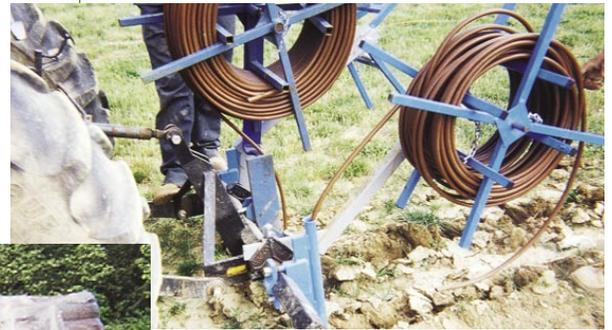
*"Techline was delivered to the job site in 1,000' coils that mounted directly onto the TLTIP insertion plow, allowing for all the drinkerline to be installed in one day."*
