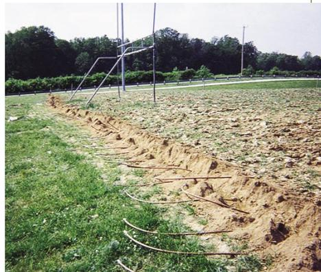
*"Techline with emitters every 18" was installed at a spacing of 18" between rows and a depth of 6". The low yield wells, which were unable to supply enough water for an overhead rotor system provided plenty of water for Techline subsurface drinkerline."*
