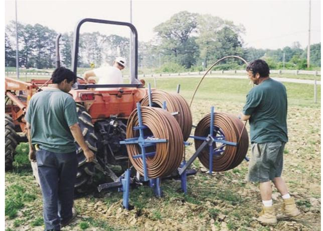
*Techline Tubing Insertion Plows were used to install the entire subsurface system in less than 10 hours.*
