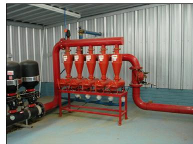
FIGURE 4 - Example of multiple small hydrocyclones working in concert.
