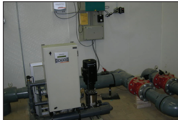
Figure 4. Fertilizer Injection system
