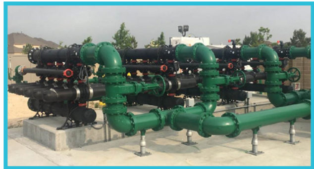
Netafim Apollo Disc-Kleen Filters (above) and Controller (bottom left).
