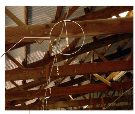
Installed in an overhead system, Netafim's SpinNet Sprinklers control dust and footing conditions in Ward's indoor riding arena used for training horses
